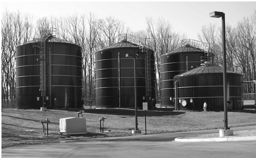
These backwash tanks are part of approximately $13 million in infrastructure improvements that ensured Jackson Township's capacity for potable water for decades to come.
